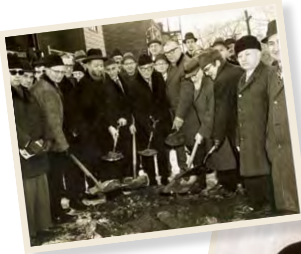
Ground-breaking at expansion of 1710 Beacon Street, Brookline building in 1968.
